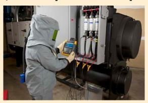
Simply hookup the voltage measurement leads and flexible current probes to the service supplying the
