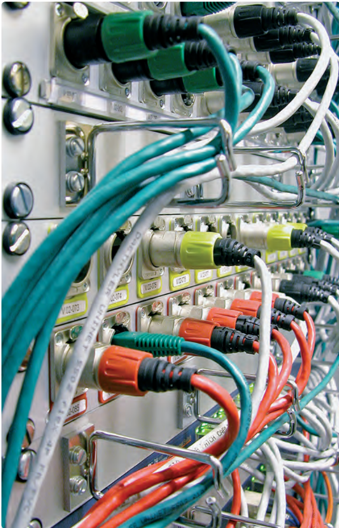
Example of etherCON RJ45 Data Connector.
