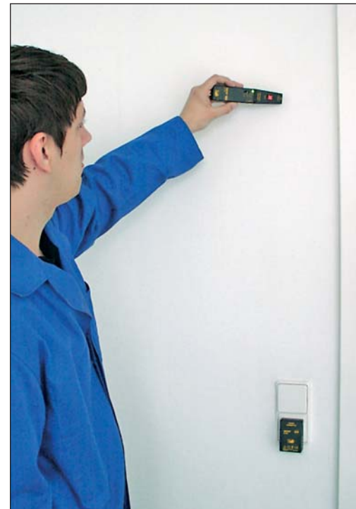
Tracing of cables
